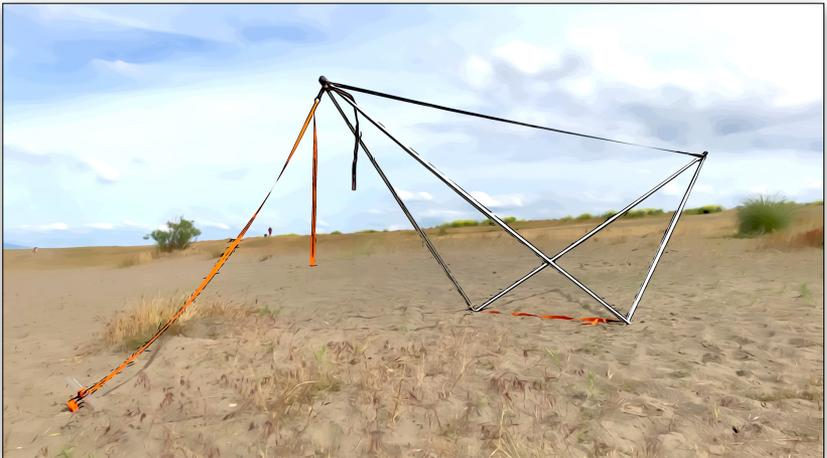
9. Attach and anchor the head end guyline. Its main purpose is to prevent the stand collapsing toward the foot side. Do **not** tighten it, now or ever. Leave it slack so the head end apex is free to move at least several inches. This allows both manual and dynamic adjustments, and avoids overloading the poles.
